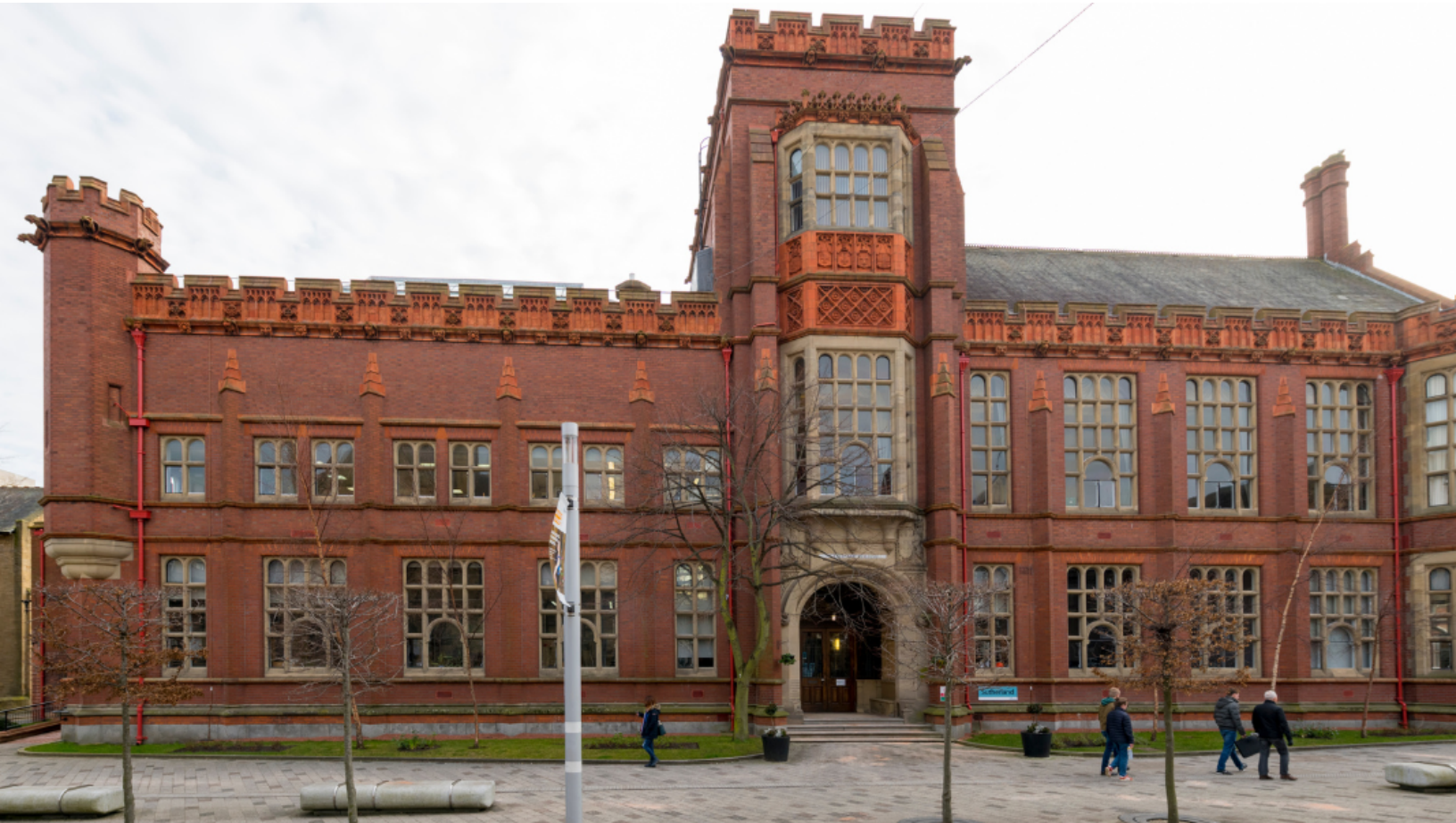
Sutherland Building at Northumbria University
